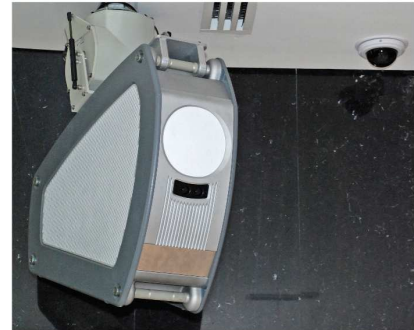
Example installation Ceiling mounted T4000 with pan-tilt.
